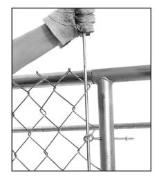
**13.** Unroll the Chain-link Fence around the frame of the kennel, being sure to keep tension on the wire by pulling the roll as you unwind it. Occasionally, it may be necessary to untangle the knuckles at the top and bottom of the roll. Keeping the tension on the roll tight will help prevent this.
