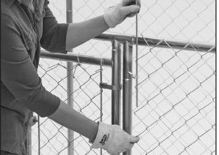
**18.** Once all excess fencing has been removed, reinsert the second Tension Rod (J) down through the Chain-link Fence and the Eyebolts on the other side of the gate, as you did in Step 12.
