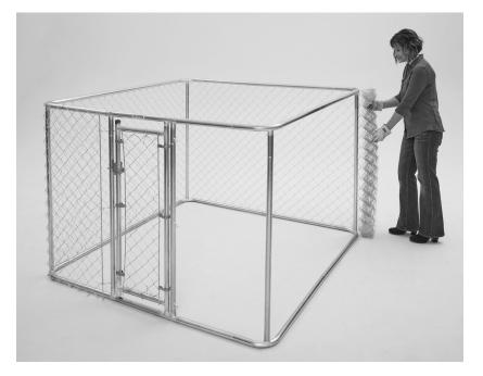
**NOTE:** As stated on page 6, with two people the fence can be fully unrolled, stretched out in its entirety, and lifted, pulled, and stretched around the perimeter one small section at a time. This will minimize bunching and tangling of the fence during application.
