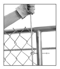
**12.** Unroll the Chain-link Fence around the frame of the kennel, being sure to keep tension on the wire by pulling the roll as you unwind it. Occasionally, it may be necessary to untangle the knuckles at the top and bottom of the roll. Keeping the tension on the roll tight will help prevent this.
