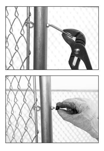
**19.** Starting at the Door, install Short Plastic Ties (Q) every two feet on the top rail, securing the Chain-Link Fence to the Top Rail of the Kennel. Do the same with the Bottom Rail, installing the ties <u>with closer</u> <u>spacing, approximately every 12 inches</u>.
