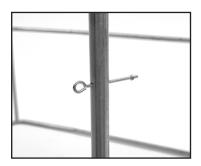
**15.** Next, stand one end of the Chain-Link Fence (L) up against the left side of the Gate frame. Starting at the top, thread the Vertical Tension Rod (J) down through the Chain-Link Fence, front/back, front/back, through each diamond, while making sure to pass <u>through</u> the eye of each Eyebolt on the way down. Thread the rod all the way through the last diamond at the bottom.
