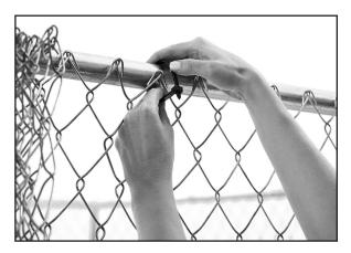
**18.** After you have unrolled the Chain-Link Fence completely around the frame, you may find that you have several extra inches of wire that extend past the last set of Eyebolts. This excess must be removed. Pull the Chain-Link Fence tightly past the Eyebolts to determine where to remove the extra fencing so that the second Tension Rod can be installed as in Step 15.
